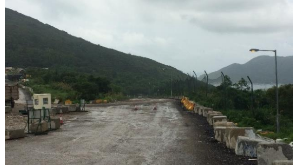
Access road and topography in South-East SENT Landfill
