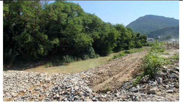
Drainage channel in TKO Area 137
