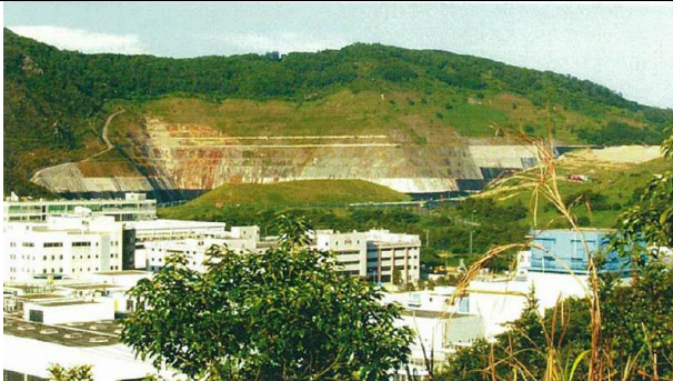
Man-made slope with shrubs and grass in SENT Landfill
